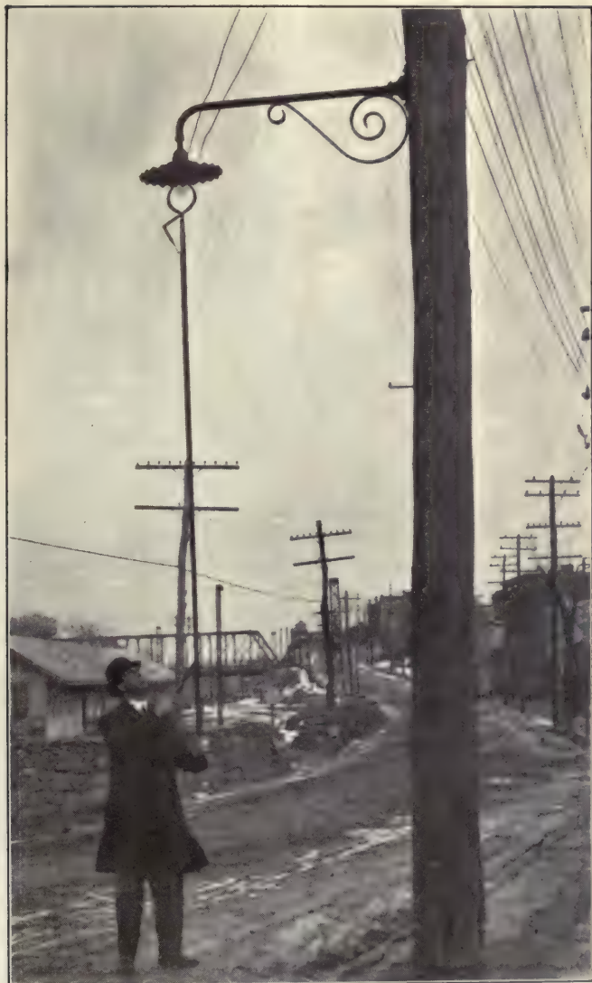
FIG. 2.—Method of using device to remove lamps from the ground.
